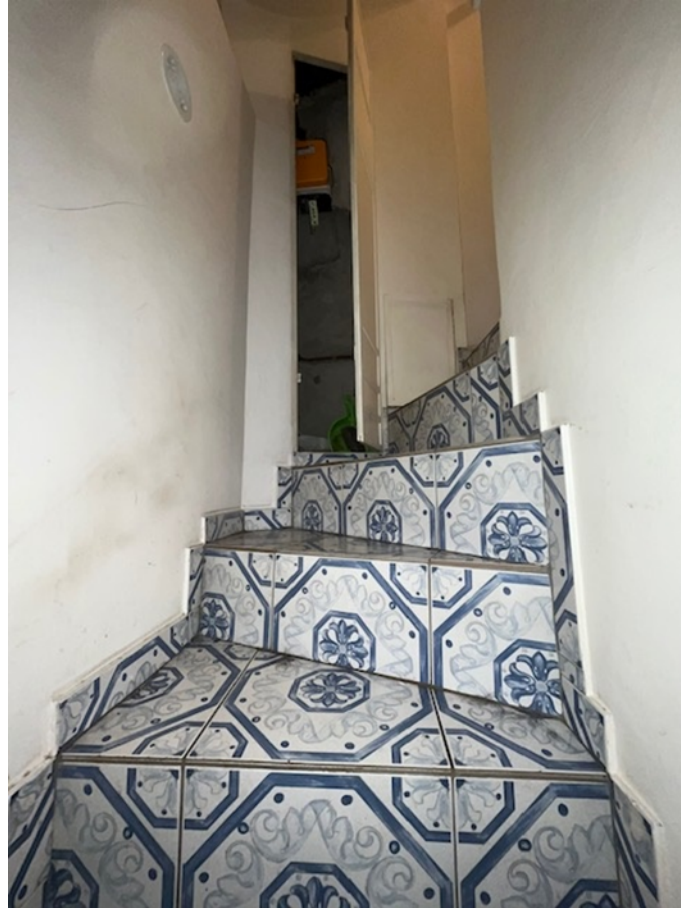
Figure 5: Example of a gas flowmeter (in yellow) with a difficult access.
